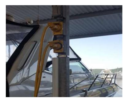
The weight of the cords combined with the movement of the boat can pull the connector resulting in a failed connection and damage to both the shore power cord and the outlet. Poor connections can result in overheating, electrical arcs and fires.
