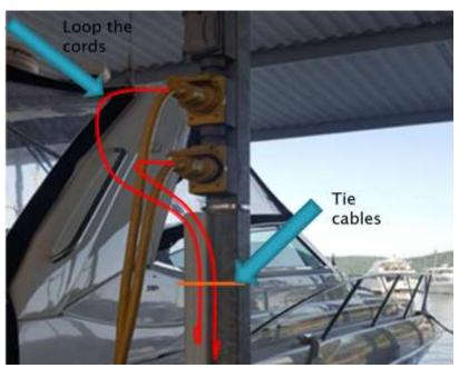
A better connection show in red would provide support for the cables so the connector not taking the weight of the cables and is isolated from vessel movements.
